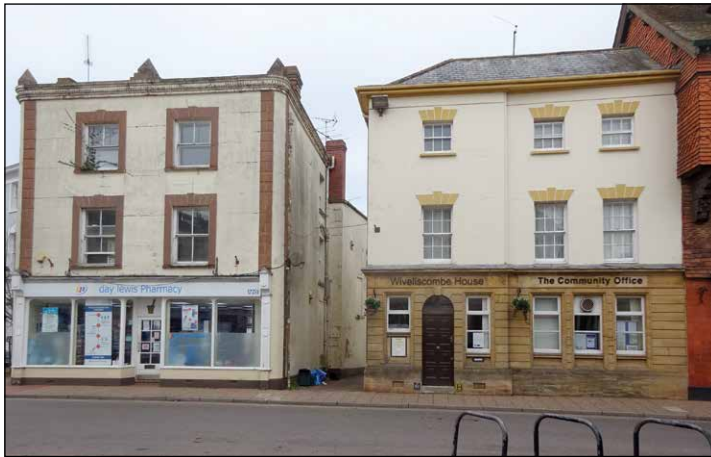
The classically styled Pharmacy and Community Office are key facilities in The Square.
