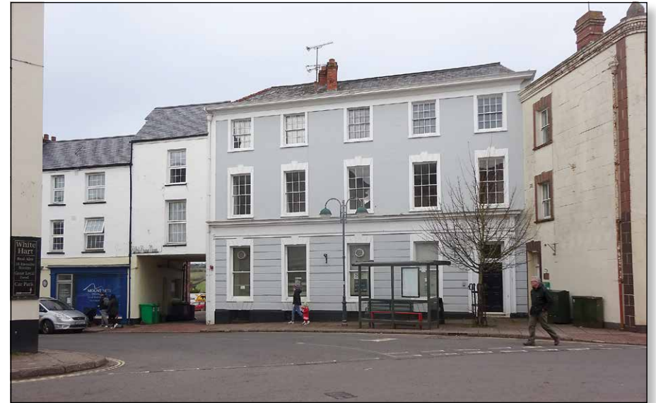
The well-maintained late Georgian former bank building maintains the formality and scale of The Square whilst making the transition to the more domestic scale of North Street.
