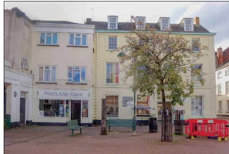
West side of The Square, with London House and the later Whelan's Café building.
